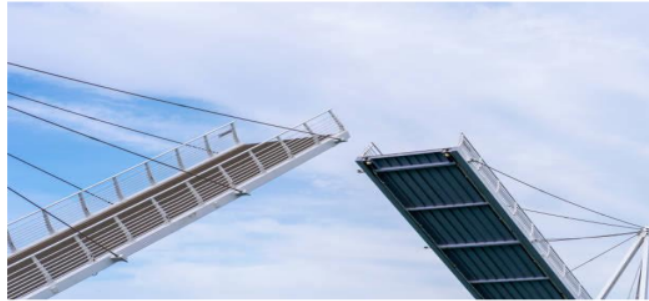
GAMBAR 2.6, Jembatan Movable Bridge/Jembatan gerak
