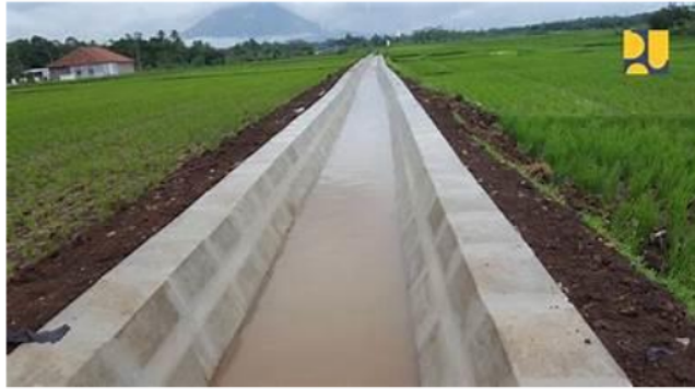
Gambar 2.20 Talud (Sumber, https://space-kd.sgp1.cdn.digitaloceanspaces.com/ )
