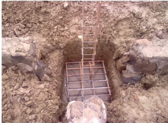
Gambar 2.1 Pondasi Dangkal (Sumber, https://3.bp.blogspot.com/ )
