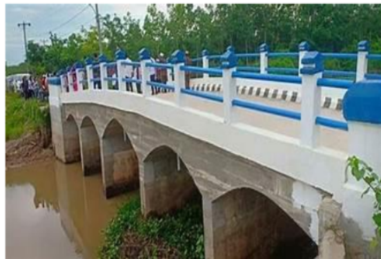
Gambar 2.16 Jembatan Beton (Sumber, https://cdn.kibrispdr.org/ )
