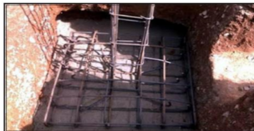
Gambar 2.2 Pondasi Foot Plate
